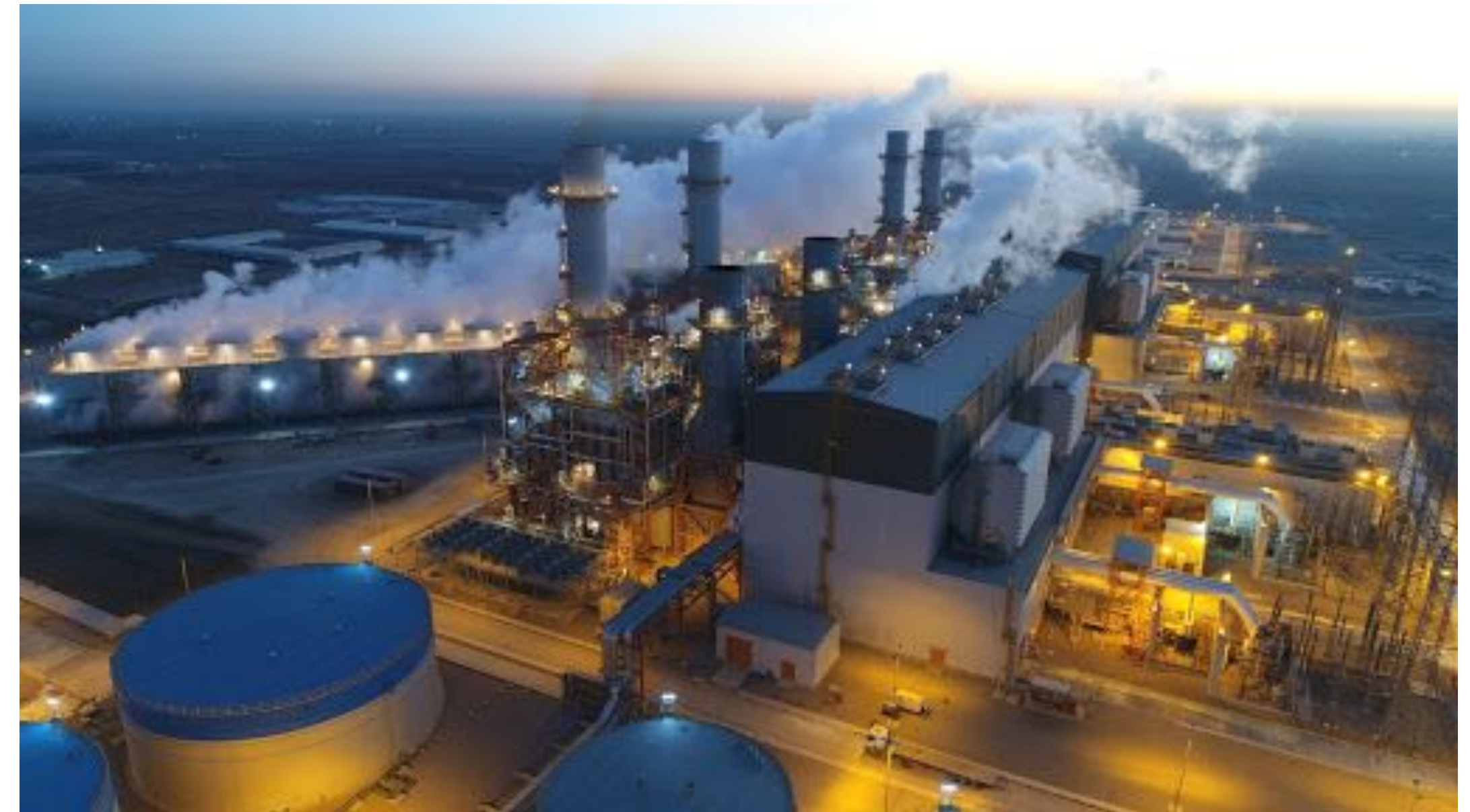
Besmaya Power Station in Baghdad (Mass Holding Group)
