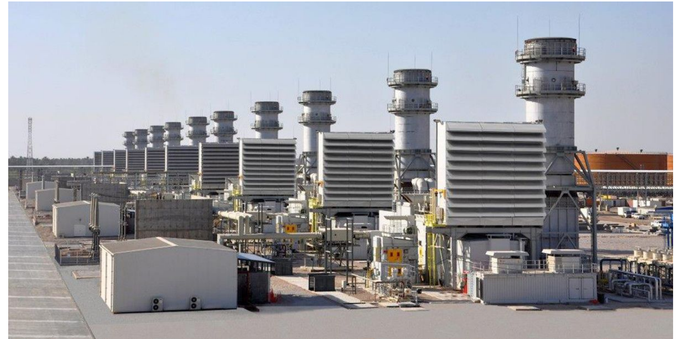
AL-KHAIRAT 10 MODULES X125 MW SIMPLE CYCLE GAS TURBINE POWER PLANT (IDOM 2014)
