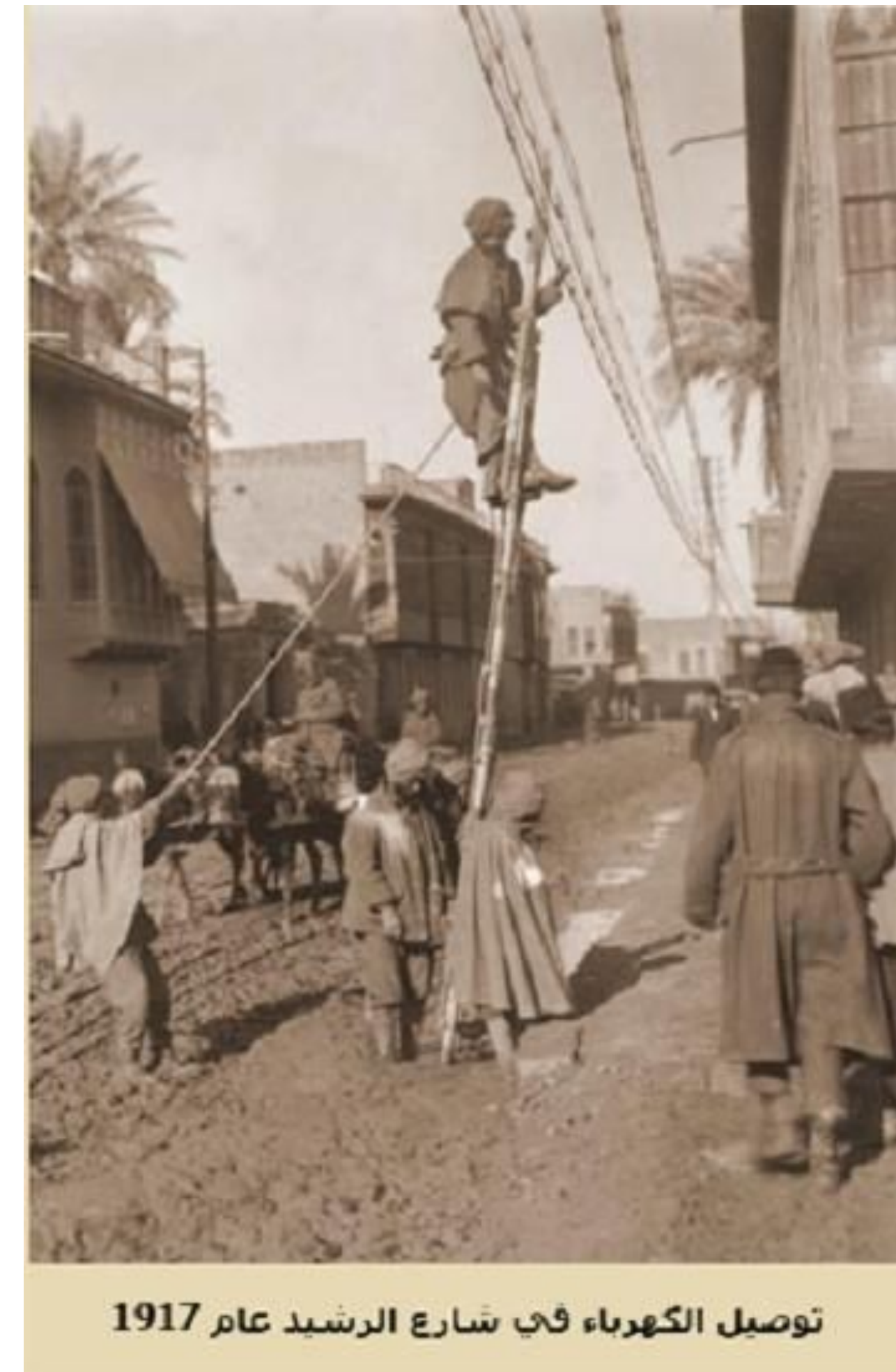
One of the earliest electrical connections in Iraq in 1917. (Al gardenia 2015)
